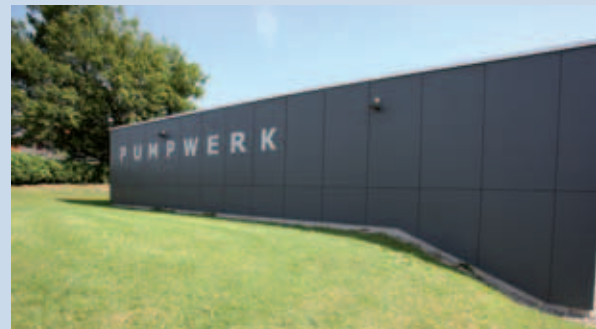
Pumpwerk in St.Margrethen
